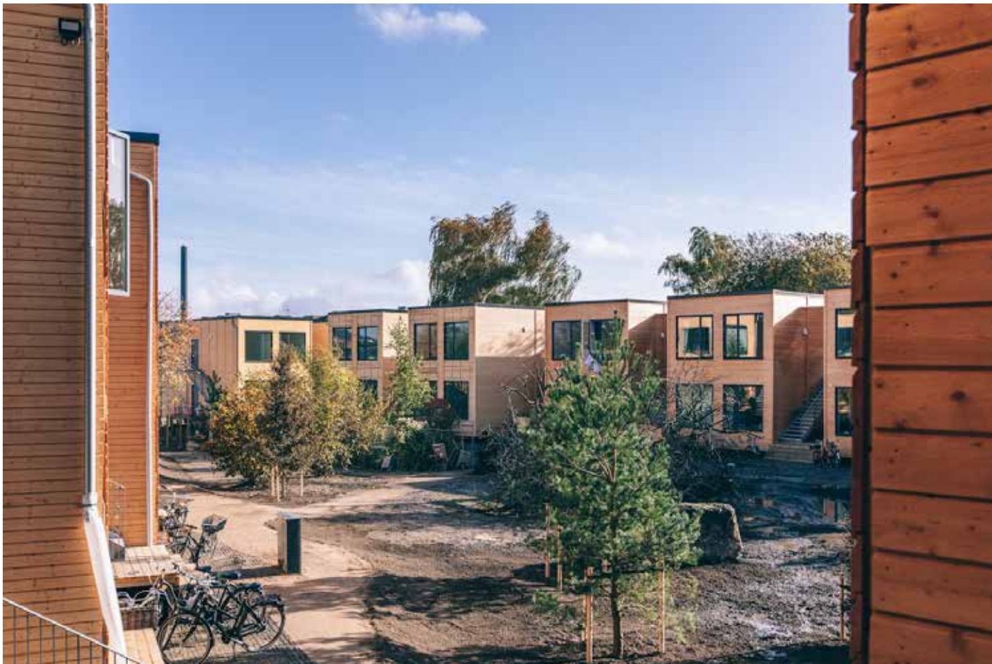
CPH VILLAGE, DENMARK
