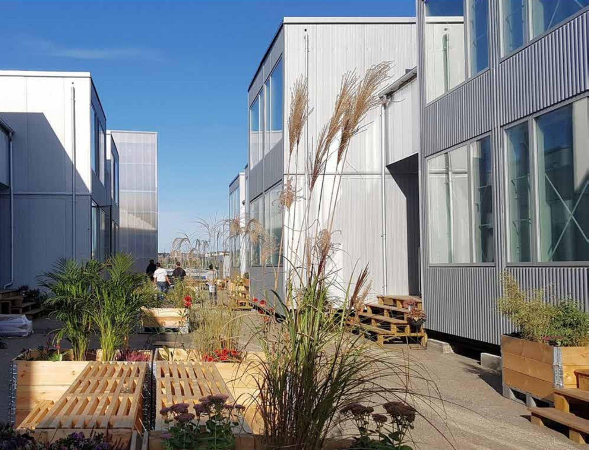
CPH VILLAGE, DENMARK
